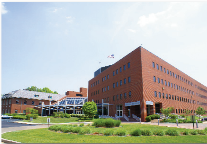
IMG World Headquarters, Indianapolis, Indiana
